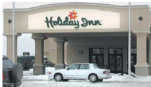
The Holiday Inn in Fargo, ND, where Capstone solved a hot water shortfall while generating an electricity dividend.
